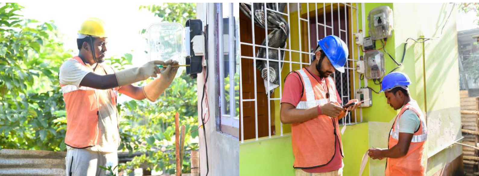
Workers installing smart meters at homes
