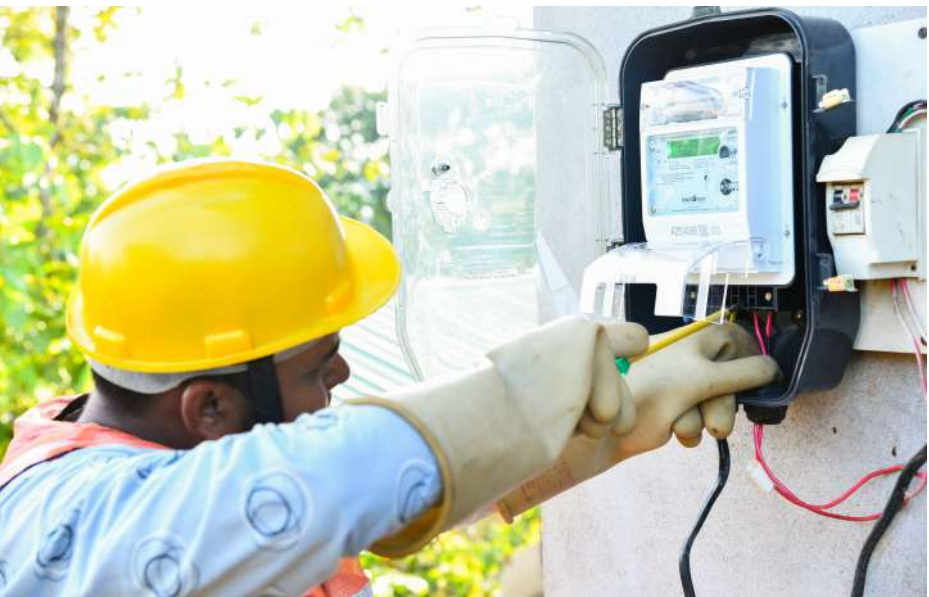
IntelliSmart workers on the field installing smart meters
