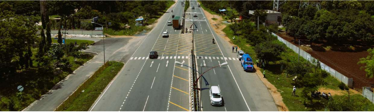
Lane markings for enhanced road safety
