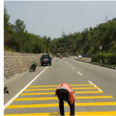
Road safety improvement work on highways
