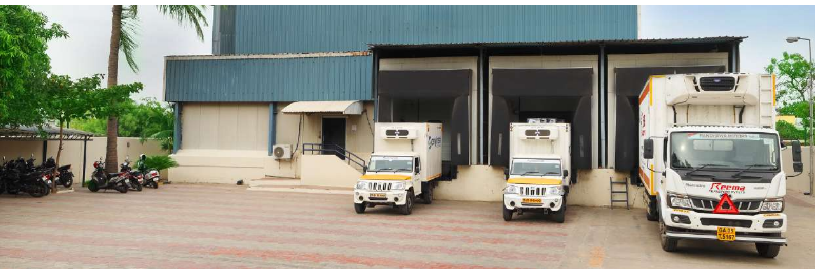
HIPL's Cold Chain Warehousing Facility
