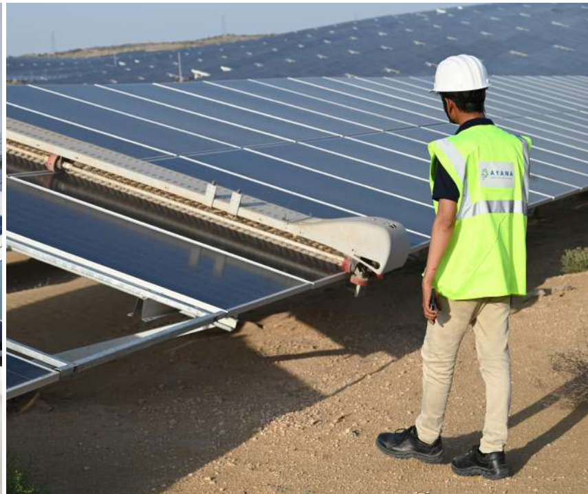
Robotic dry cleaning technology being used to clean solar panels at one of Ayana's solar power sites
